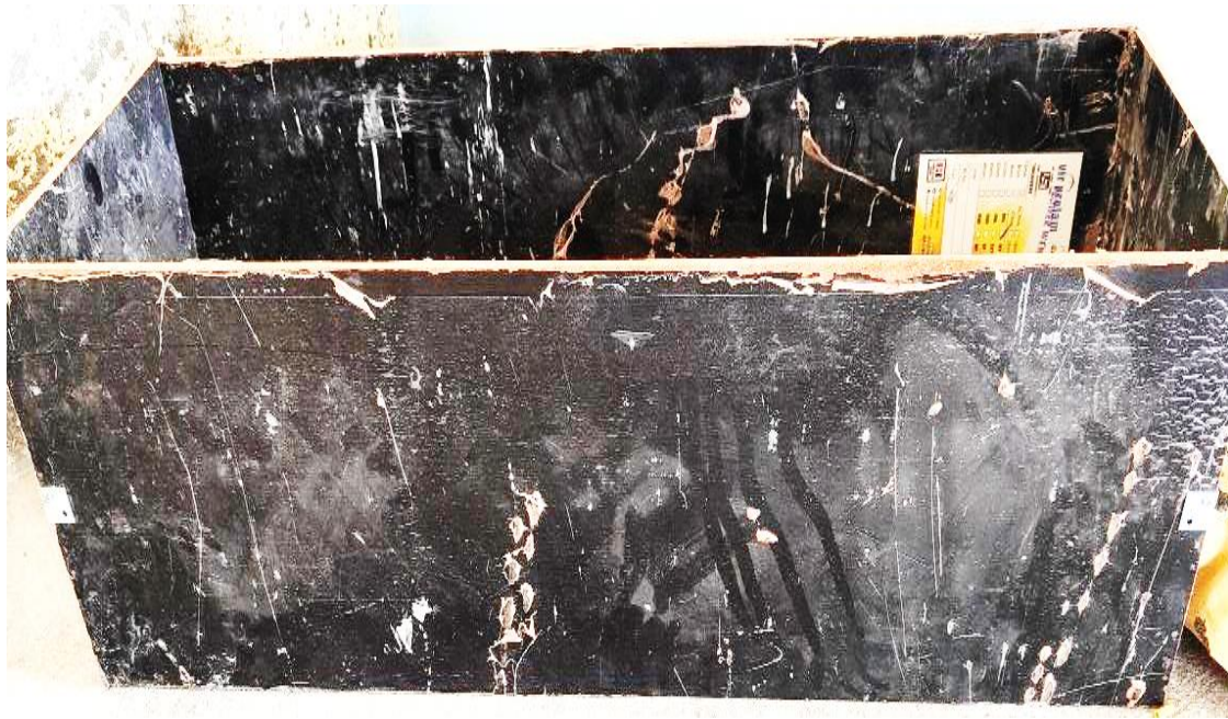
Fig.3.1 Plywood Mould for Precast wall Slab
