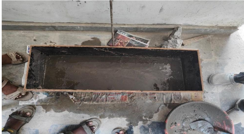
Fig.3.3 Concreting of Precast Wall Slab
